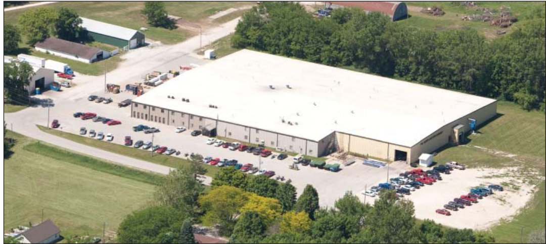
Chantland-MHS' 90,000-square-foot manufacturing facility and headquarters. Aerial photo supplied by Chantland-MHS.
