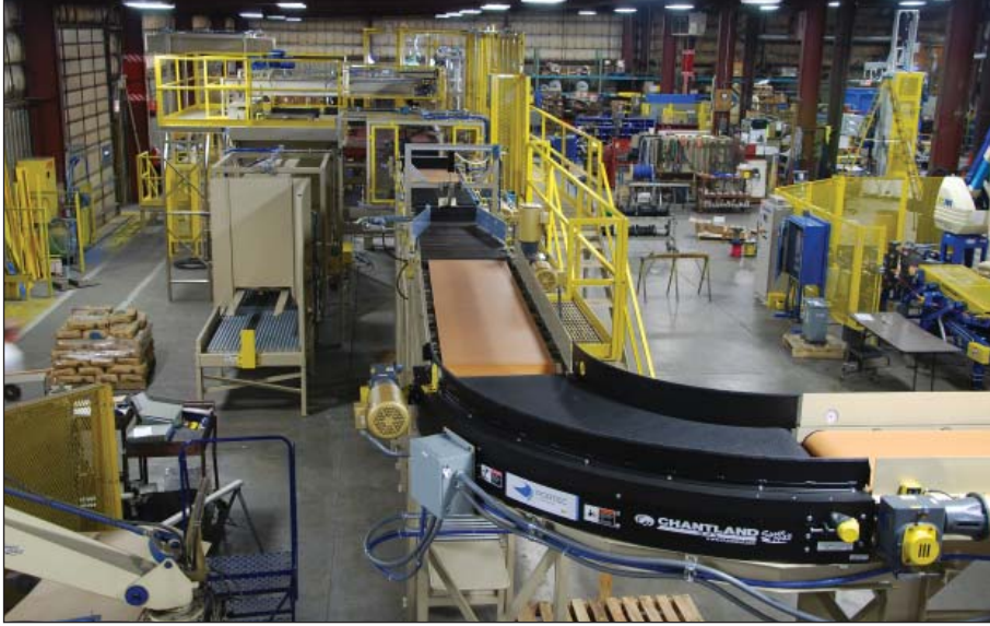
Conventional and robotic bag palletizers fully assembled, hard-wired, and plumbed in preparation of factory acceptance tests.
