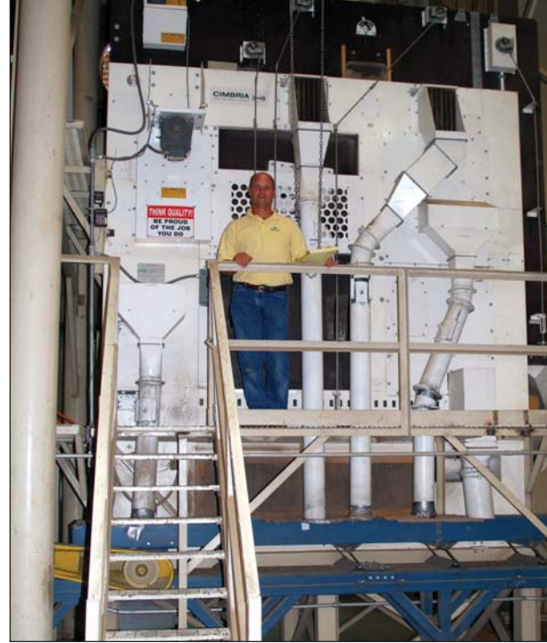
General Manager Marty Eaton with a Cimbria Delta 108 air screen installed in 2004.
